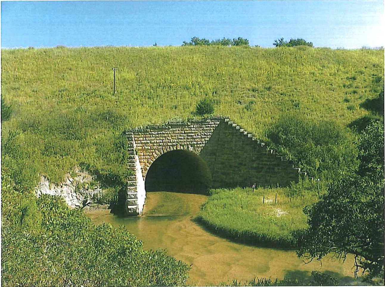
Above: The largest stone arch culvert on the Cowboy Line is No. 437 located three miles west of Johnstown. This culvert was built in 1903 for Plum Creek and has a massive opening of 32 feet and a length of 232 feet. — Jerry Penry photo
