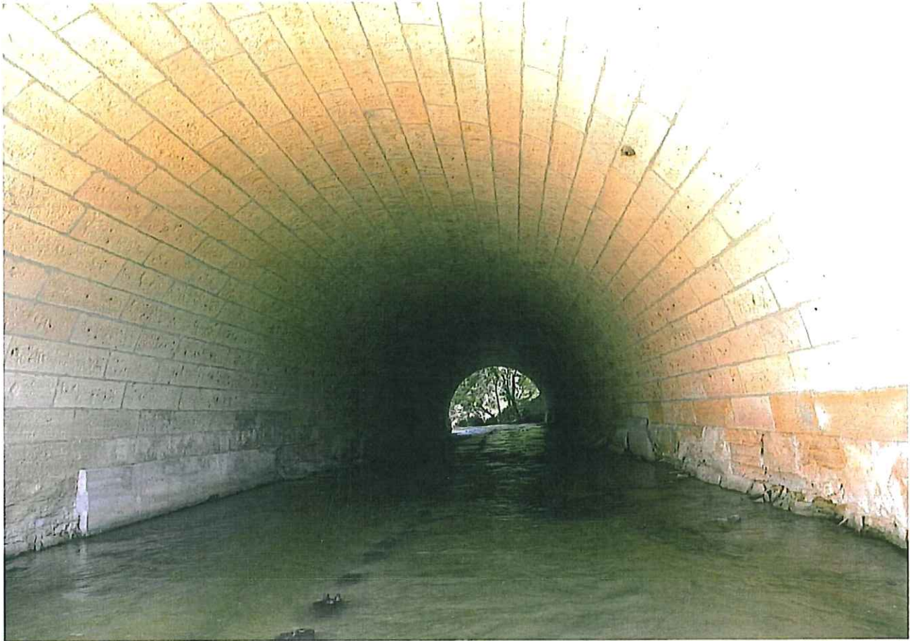
Above: The stubs of timber piling can still be seen coming up from the floor in Culvert 437 that was built in 1903. These pilings supported the wooden framework while the culvert was being built. — Jerry Penry photo
