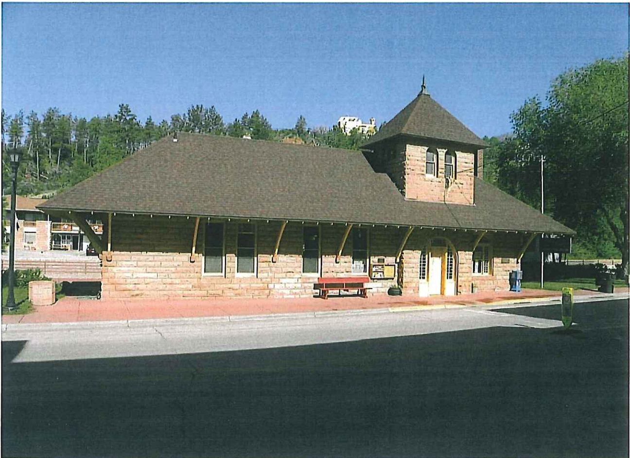
Above: The station at Hot Springs, South Dakota, was built in 1891 from native sandstone from a nearby quarry. It is believed this same quarry supplied the stone for most of the stone arch culverts built by Charles A. Berg. — Jerry Penry photo
