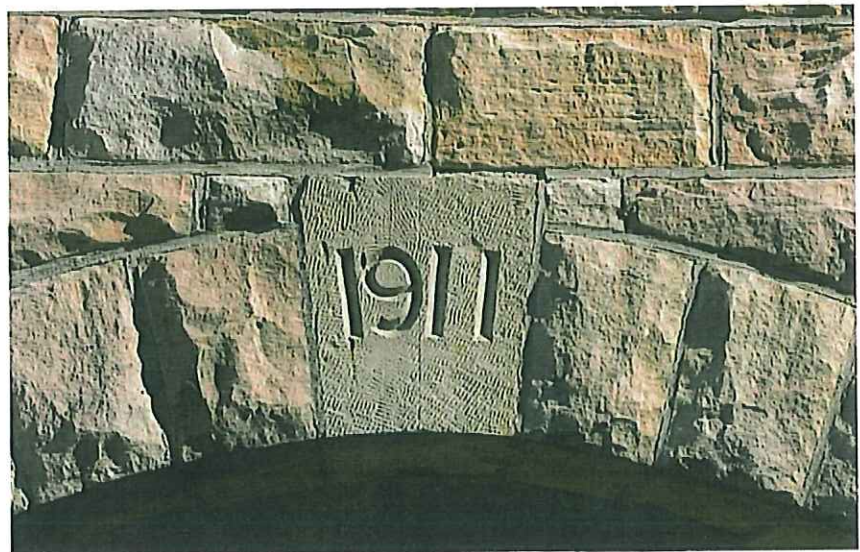
Above and right: The keystone for Culvert 439 located six miles west of Johnstown is marked with the year and Berg's initials. The keystone on Culvert 622 is marked for the year only. It is a second 10-foot structure added to an existing structure of the same size that was built in 1898 located 4.5 miles west of Hay Springs. — Jerry Penry photos
